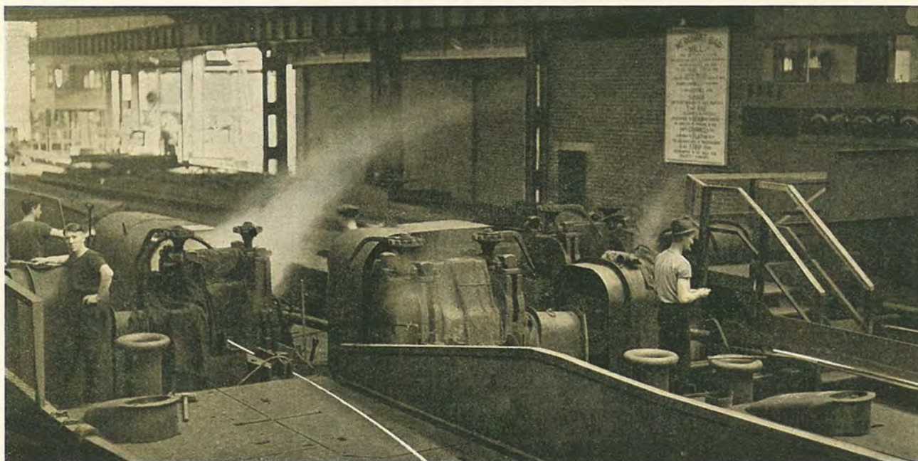
CONTINUOUS BAR AND STRIP MILL—FINISHING STANDS.
