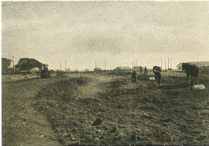
Area looking towards Lysaghts and Rylands Works during the process of levelling up.
