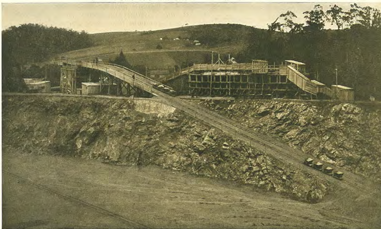
MELROSE QUARRY, SHOWING INCLINE TO CRUSHER BIN.
