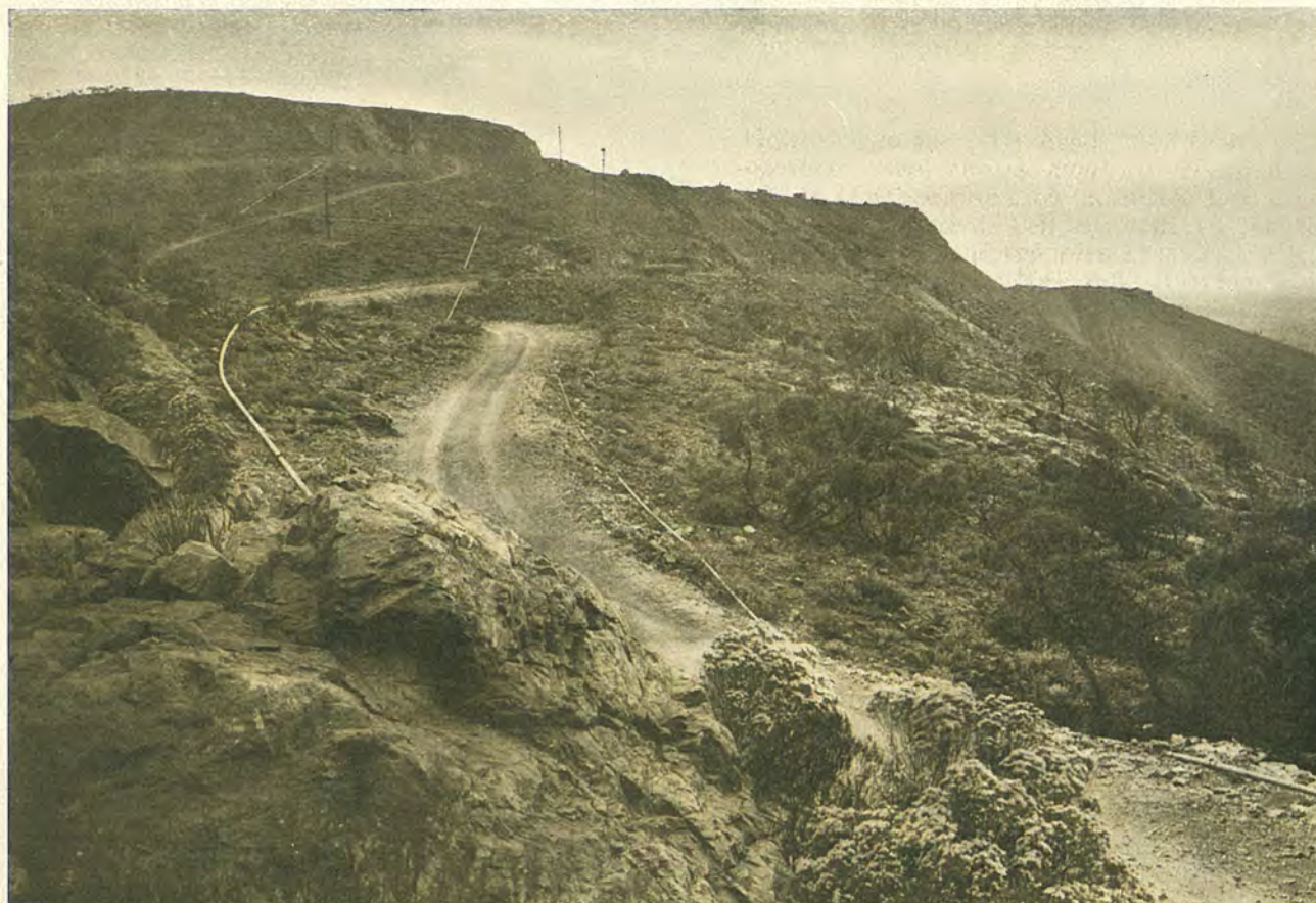
IRON MONARCH BENCHES E AND A FACES FROM SUB-STATION.
