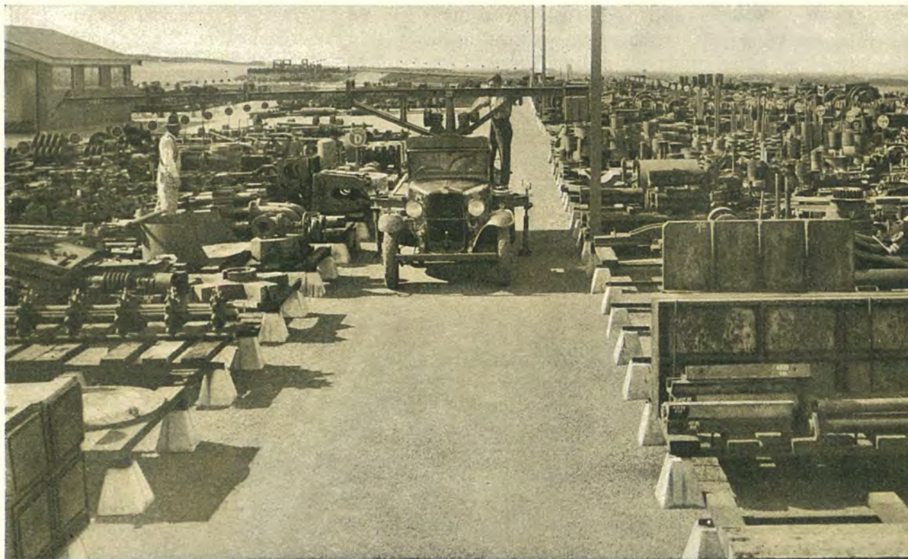
Fig. 7. STORAGE OF HEAVY SPARES, ETC., AT THE STEEL WORKS.
