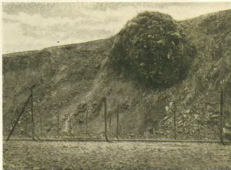
BLASTING SIX TOP AND BENCH HOLES AT IRON KNOB.
