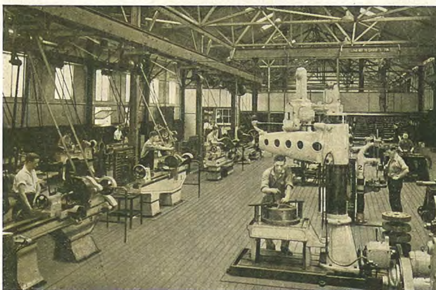
GENERAL VIEW OF MACHINE SHOP.
