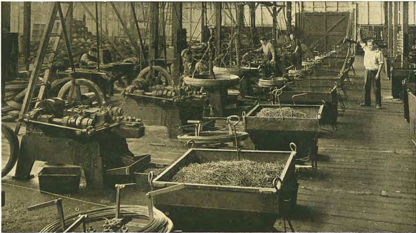
A BATTERY OF NAIL MACHINES AT WORK.
