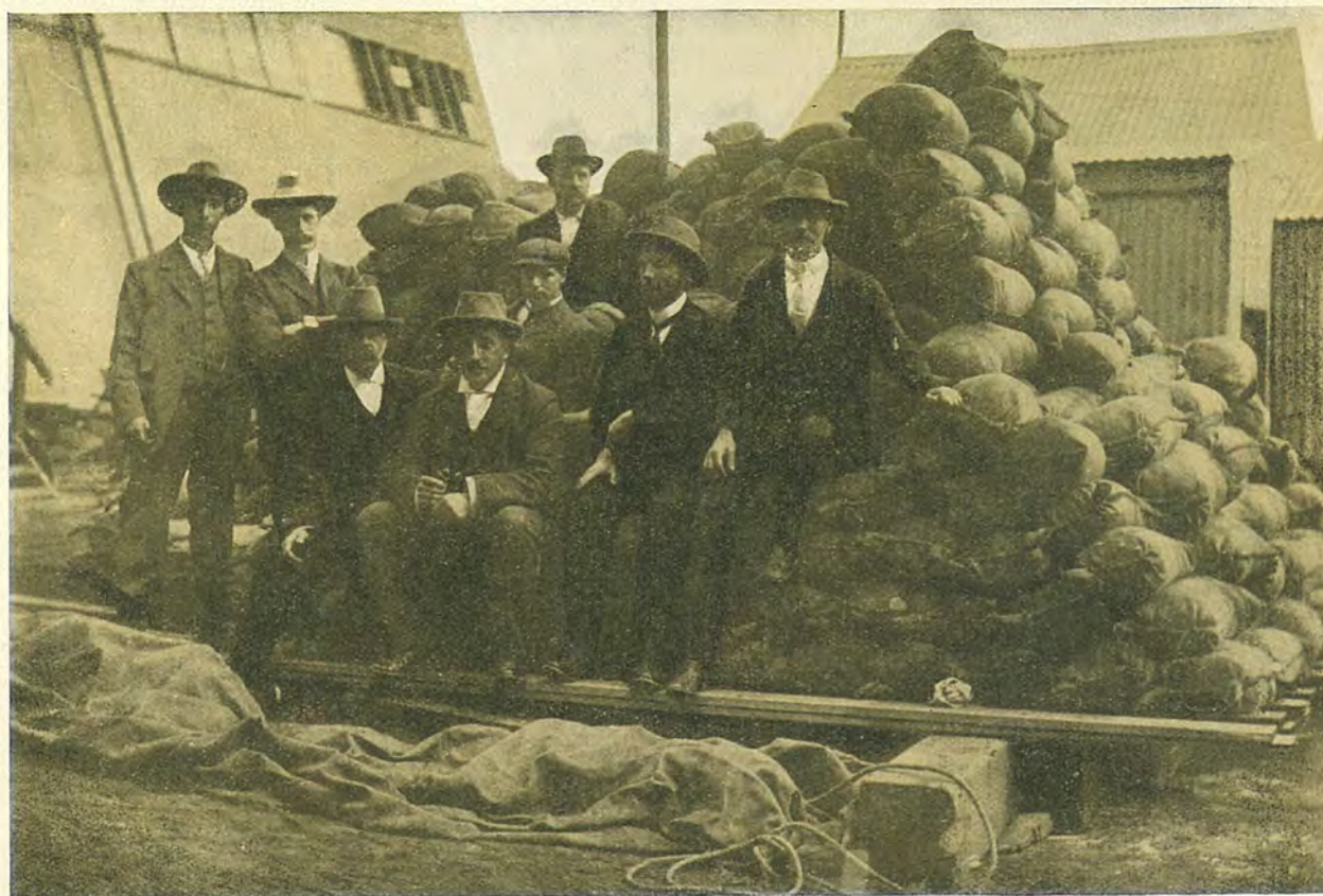
THE FIRST FIFTY TONS OF CONCENTRATES PRODUCED AFTER THE DISCOVERY OF THE FLOTATION PROCESS AT BROKEN HILL, IN 1903.
