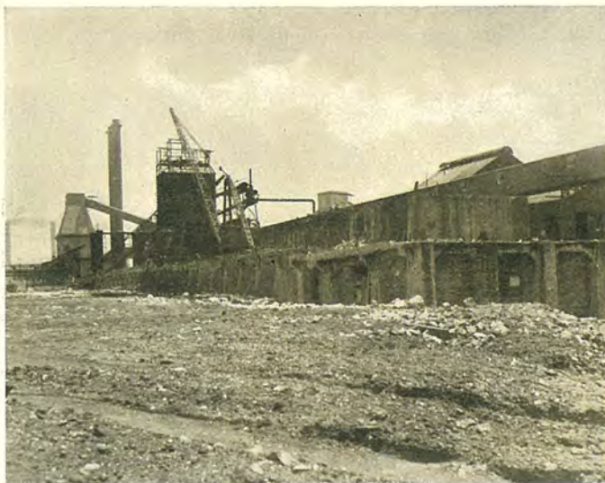
The old Semet-Solvay Coke Ovens in process of demolition.
