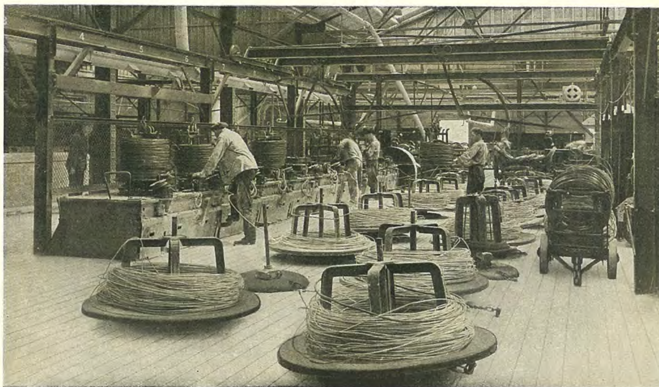
WIRE DRAWING MACHINES. FOR HEAVY WIRE. DOUBLE DRAFT PROCESS.
