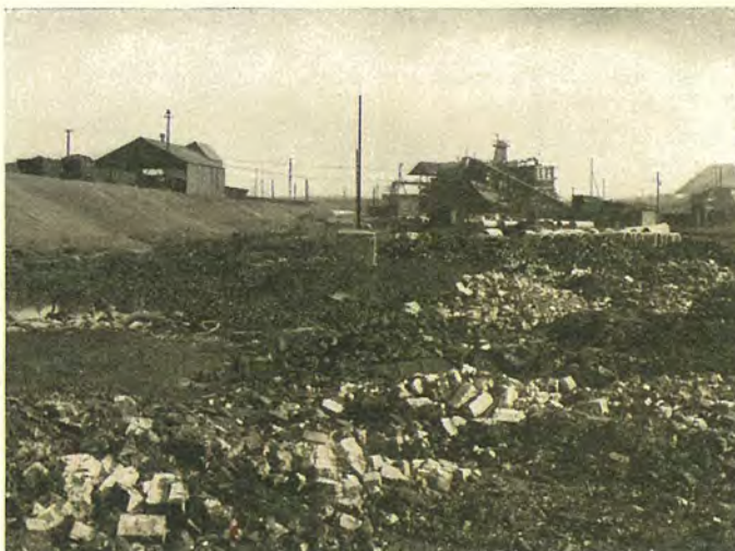
Portion of old swamps being filled with refuse prior to levelling.
