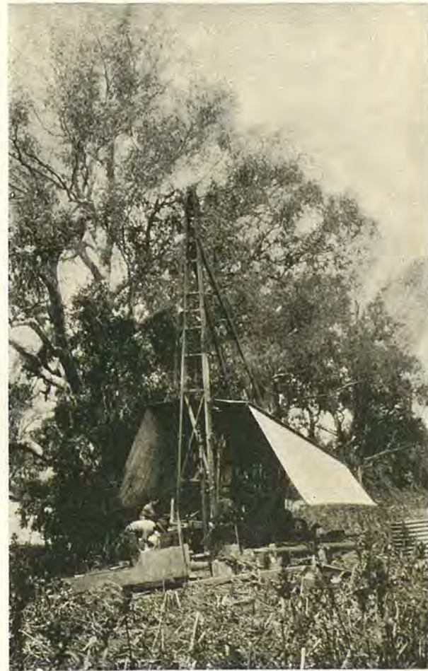
TESTING BY PERCUSSION DRILL.
