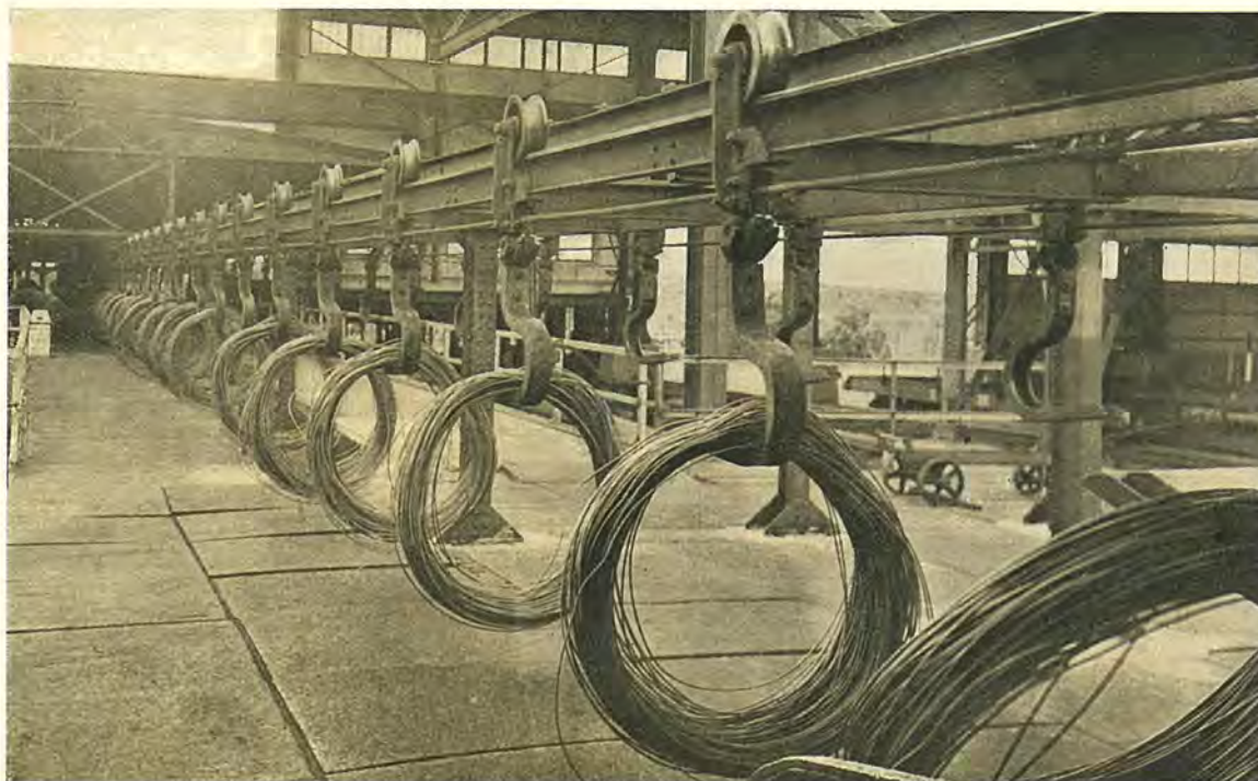
ROD MILL COOLING CONVEYOR.
