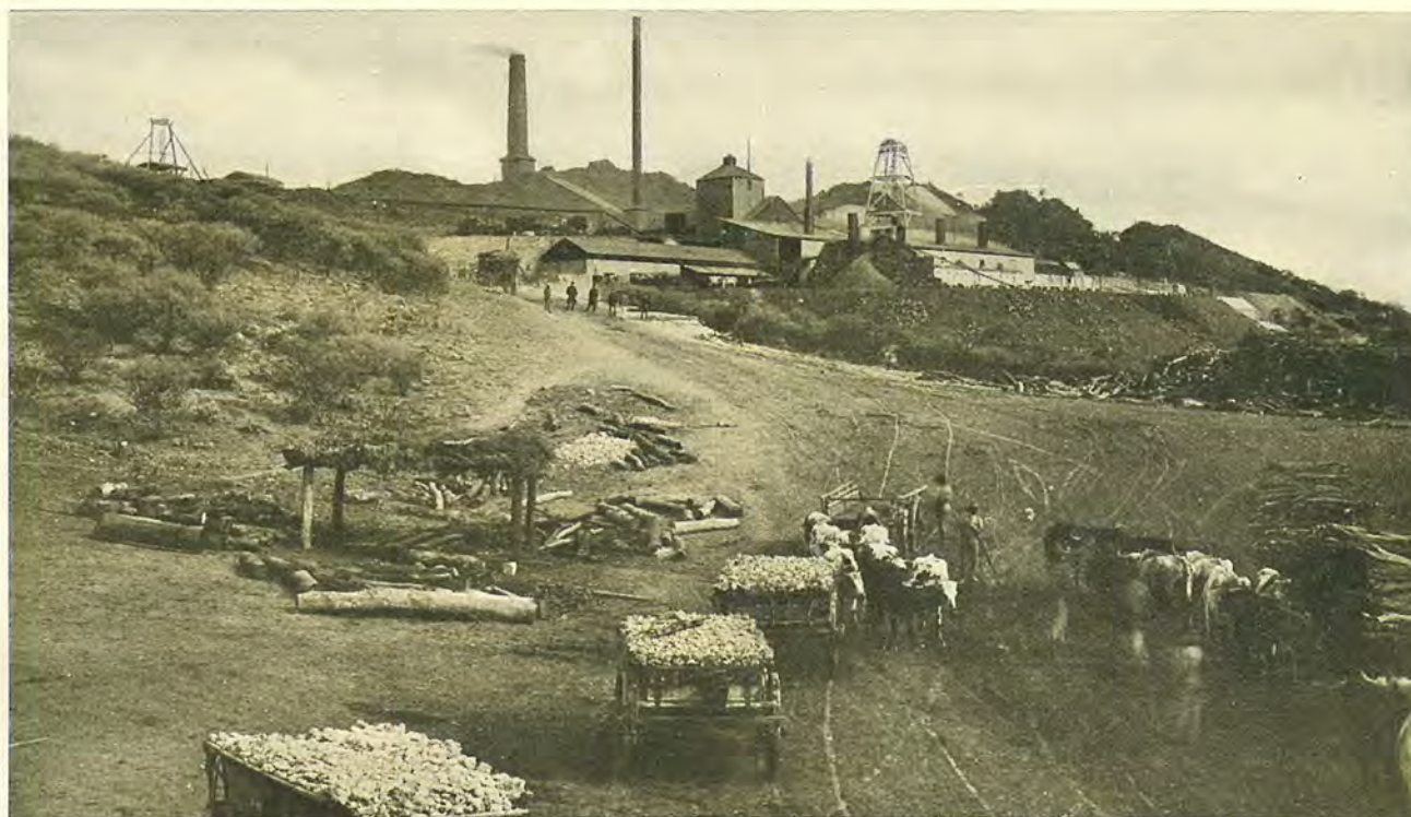
OLD 30-TON SMELTERS ABOUT 1887.
