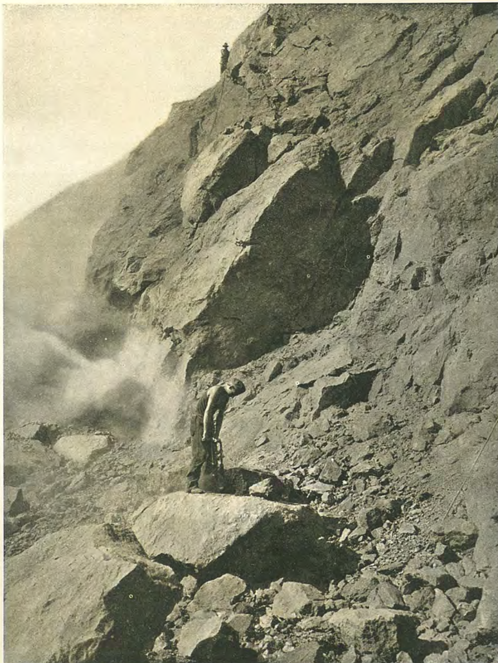
DRILLING BOULDERS FOR BLASTING, BENCH E.
