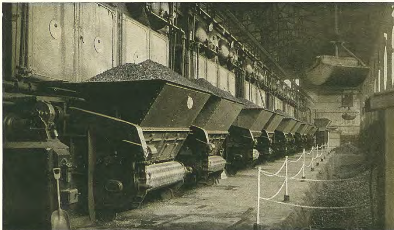
MAIN MILL BOILER PLANT.
