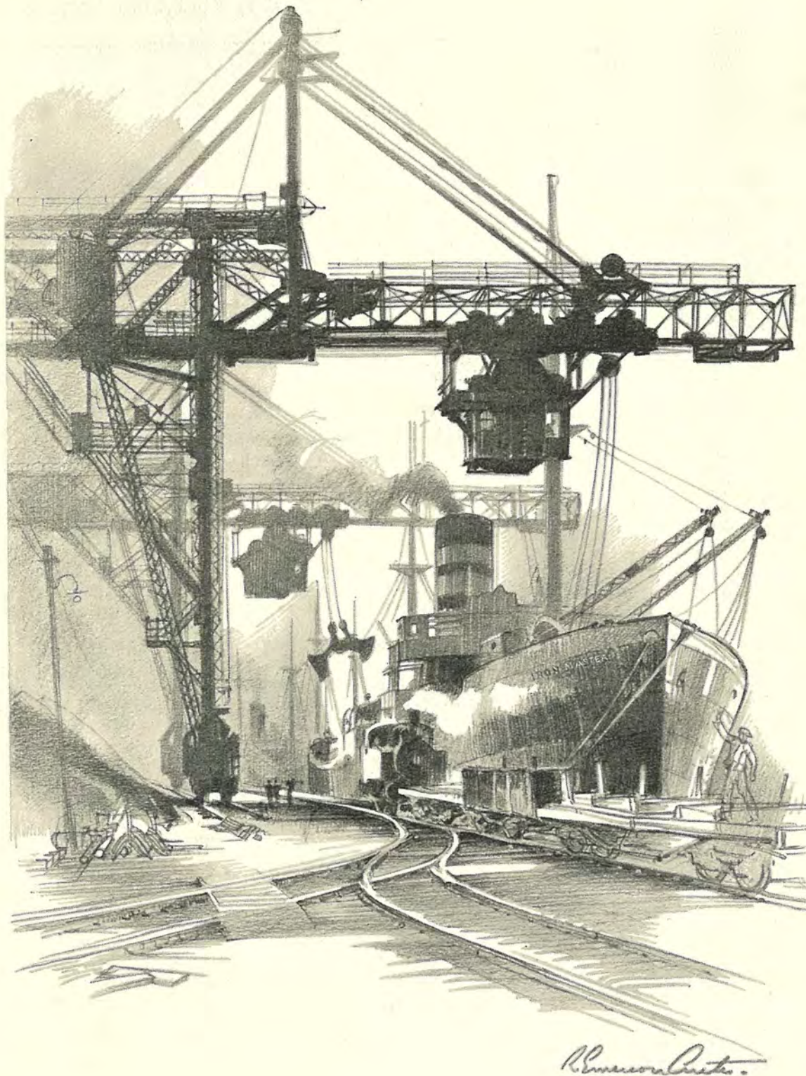
STEEL WORKS WHARF—DISCHARGING ORE.
