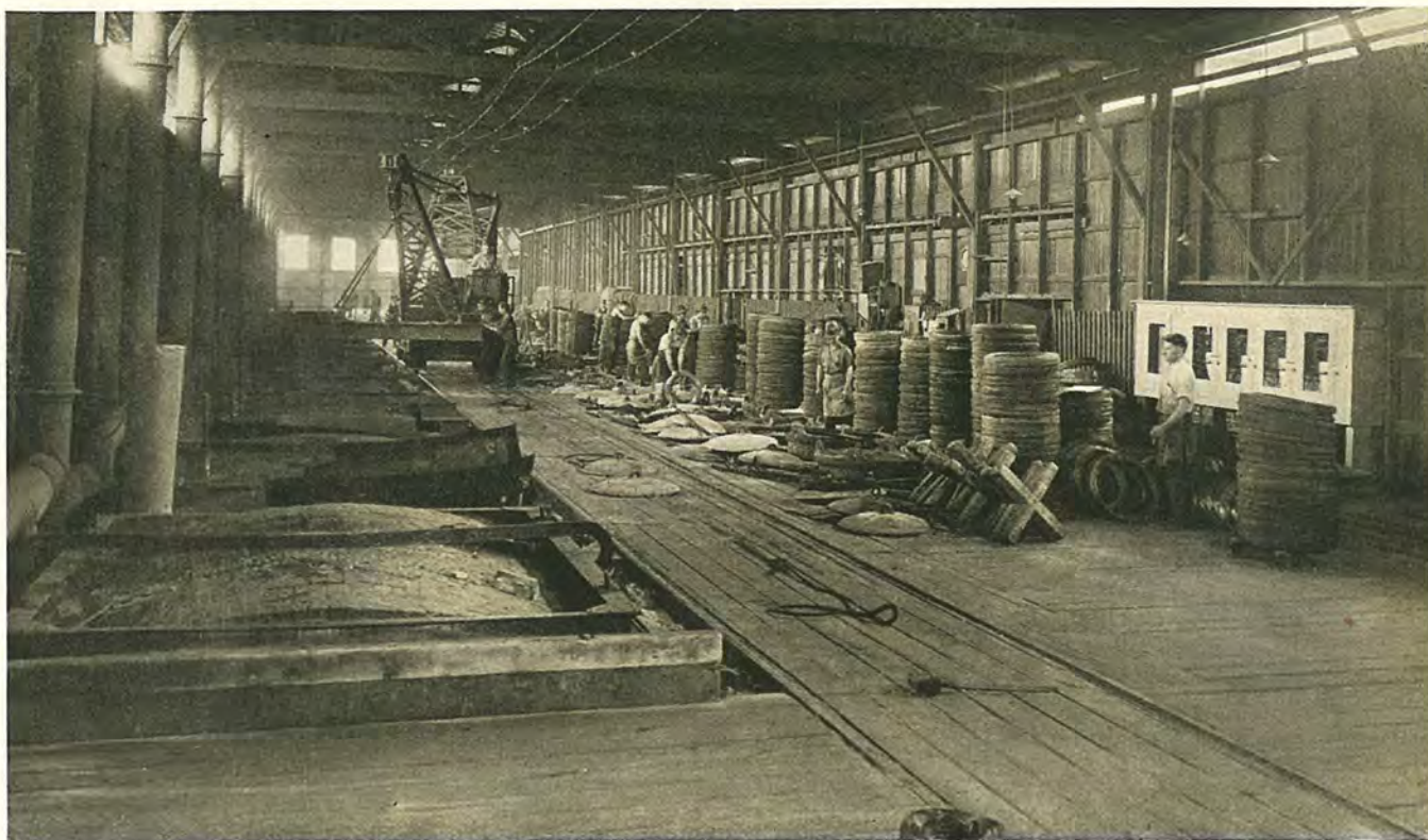
ANNEALING SHOP FOR HEAT TREATMENT OF WIRE.
