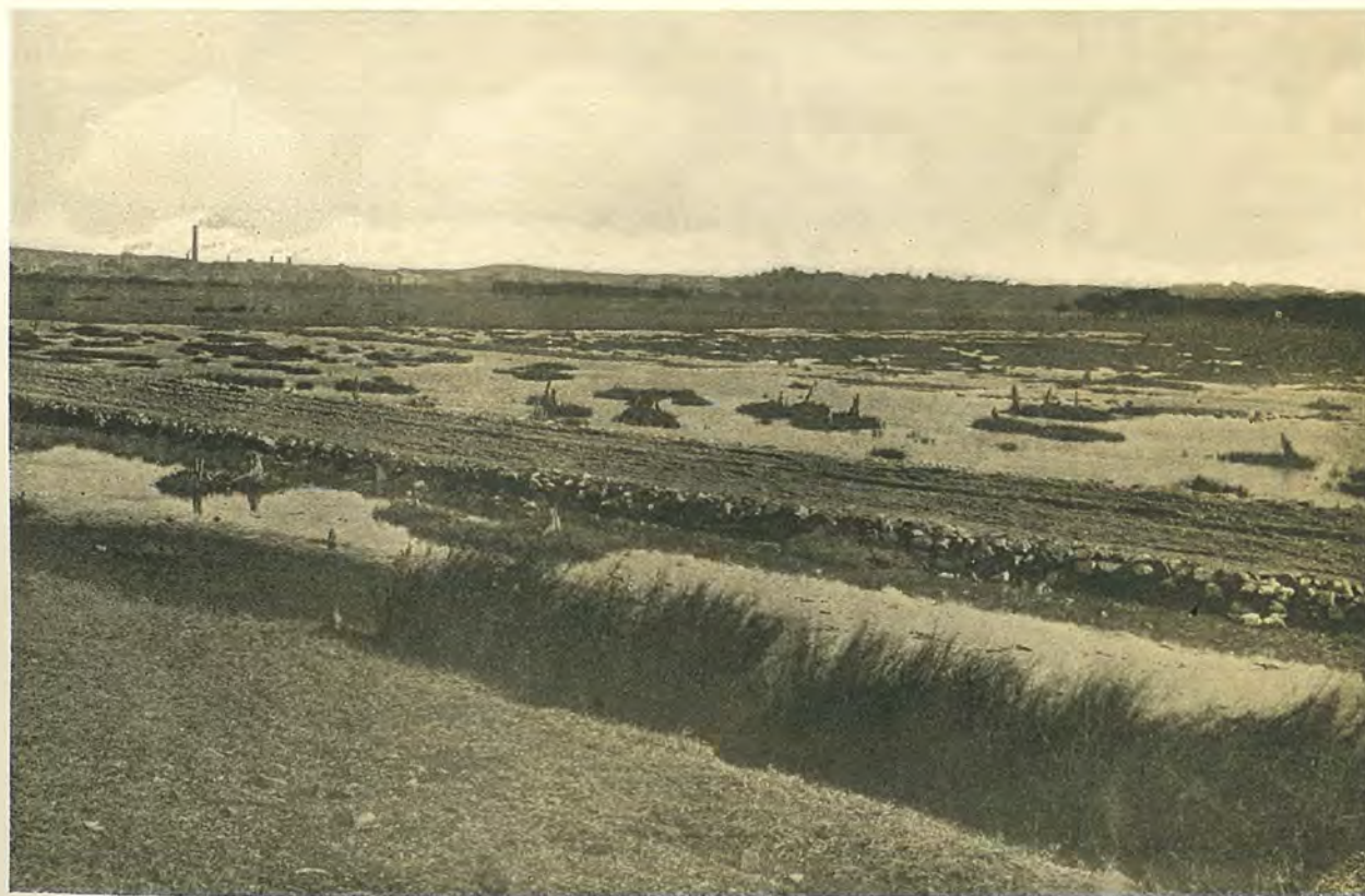
PORT WARATAH SWAMP IN 1913—WHERE THE STEEL WORKS NOW STAND.
