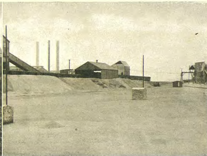
The same sector after levelling and treatment with ashes, tar spraying and blast furnace slag.
