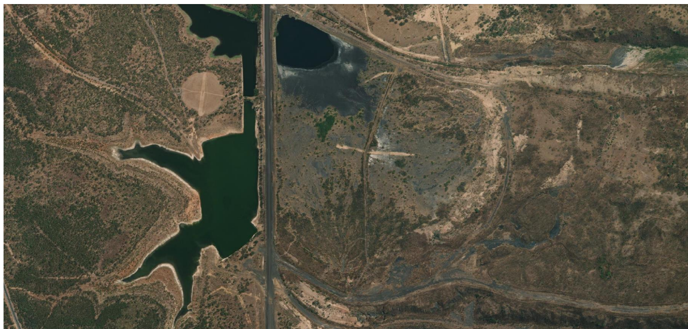
Old Tailings Dam, 2025
