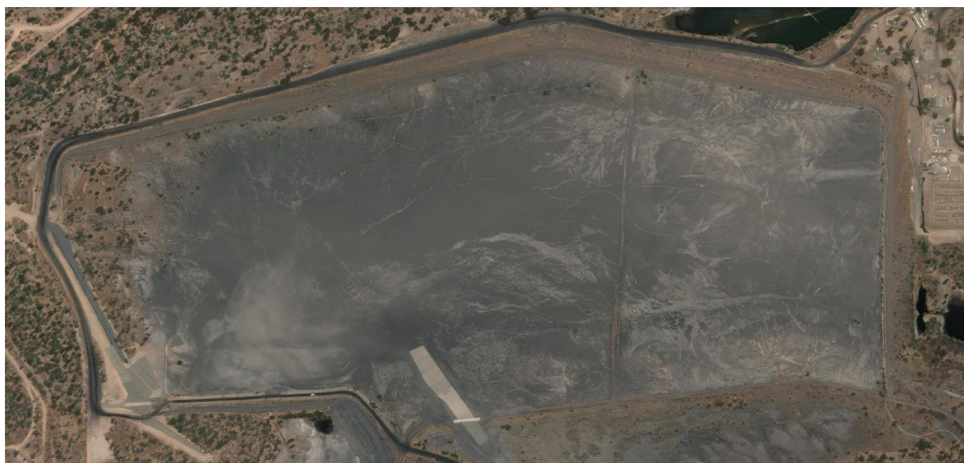
Airfield Tailings Dam, 2025
