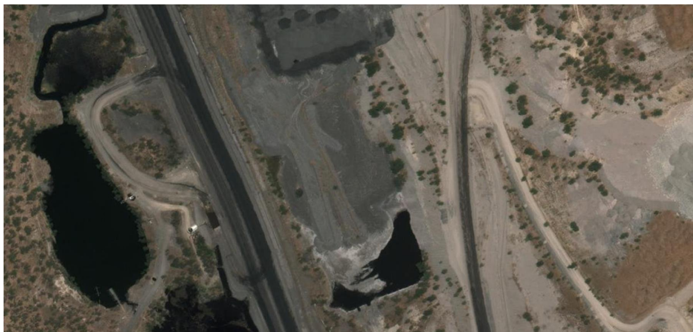
Ramp 2 North TSF, 2025
